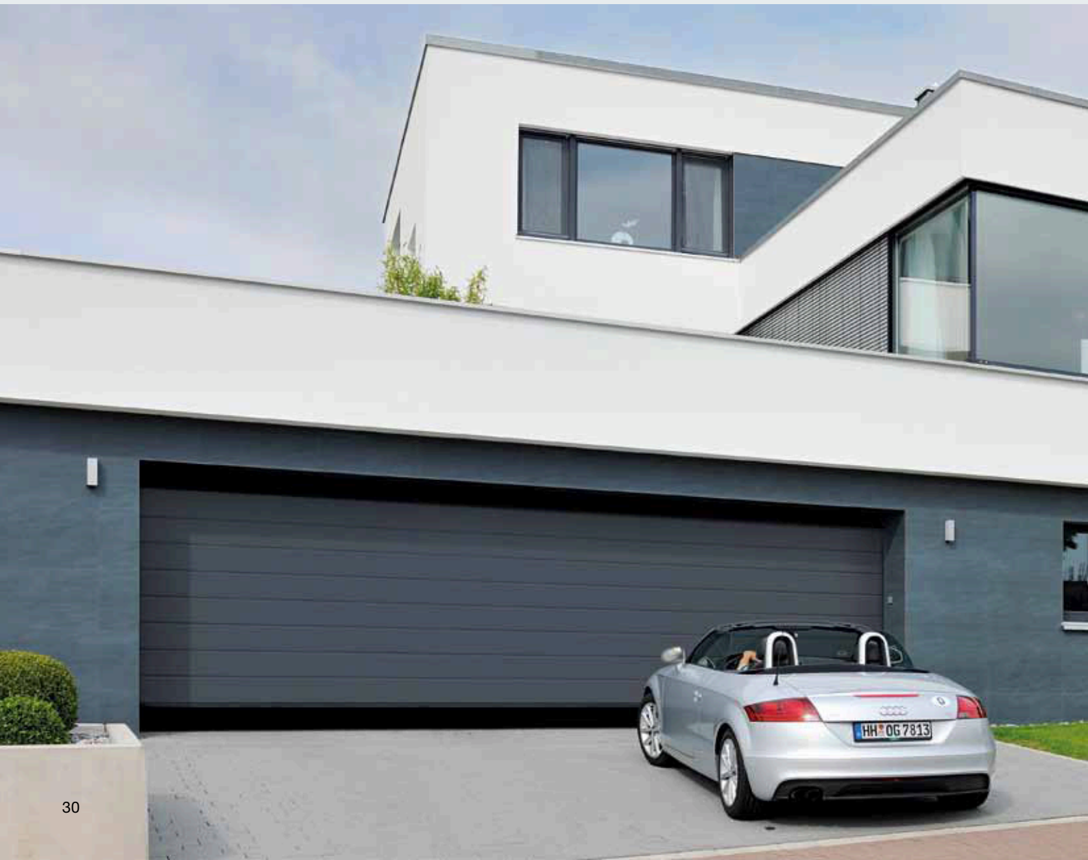
M-ribbed with the surface finish Decograin Titan Metallic CH 703
